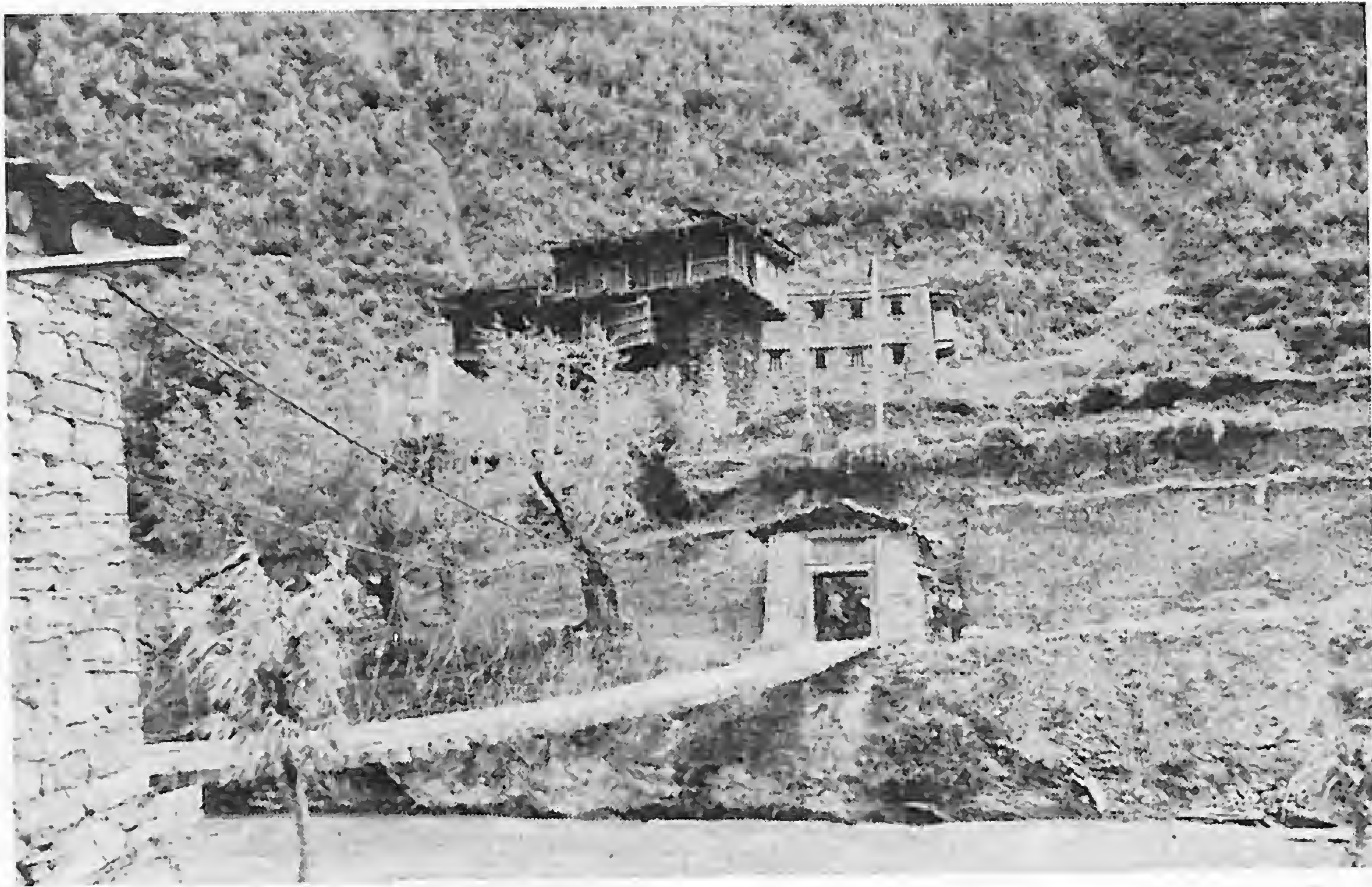
New suspension bridge to Maerhkang.
